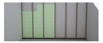
Apply the plastic mesh tape in the gypsum boards jointing lines and grouting
