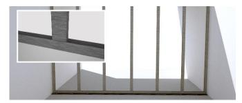
Cover the insulation layer by screwing the second gypsum boards on the metal studs
