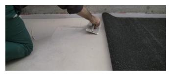
Spread the bi-component concrete glue, layer the ceramic tiles over the adhesive glue
