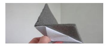
Insulate the acute corners with the Profile strip by cutting it as shown in the drawing
