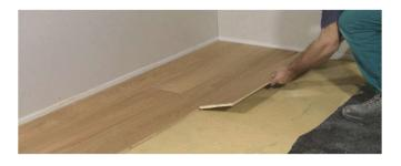
Install the acoustic mat with dimpled side facing down
