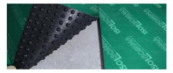
Seal the joints between panels with Stik tape.
