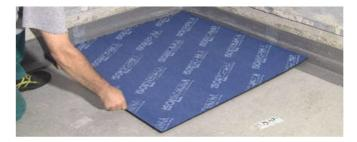
Cut the panels on the underside using a knife
