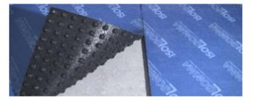
Seal the joints between panels with Stik tape.
