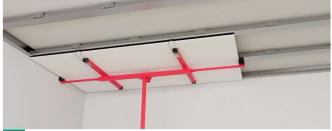
Apply the plastic mesh tape in the gypsum boards jointing lines and grouting
