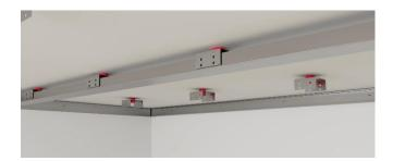
5 Fix the panel to the metal frame with gypsumboard's screws. Apply FYBRO panels if necessary
