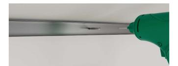
Fix the metal stud to the acoustic bracket
