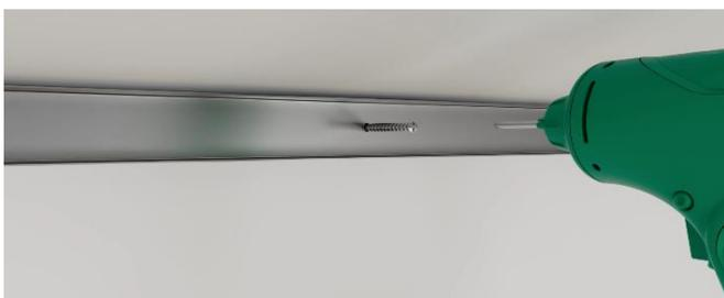
**2** Drill the ceiling and fix the acoustic bracket REDFIX C, with spacing based on the load and the type of floor
