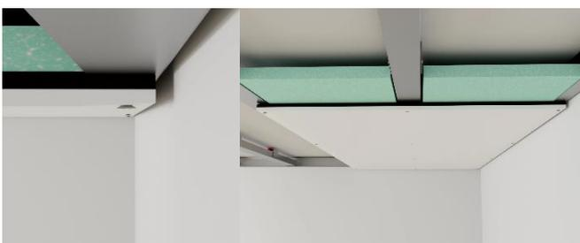
**6** Apply the plastic mesh tape in the gypsum boards jointing lines and grouting
