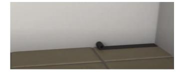
Lay points of a gypsum-based glue on the ground panel or use a low-expansion polyurethane glue
