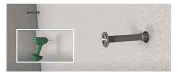
Fix the second gypsum board with the glue and/or appropriate screws
