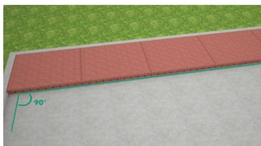
Install the first row of tiles to the edge of the other side checking for proper alignment and perpendicularity
