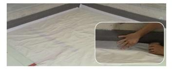
Apply the finishing on top of the screed and cut the exceeding edging strip only at the end.
