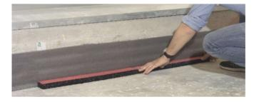
Seal any gaps higher than 2 mm between panels, using the Stik tape.
