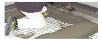
Install Highmat on the whole surface, staggered between two adjacent rows.
