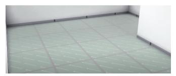
Apply the finishing on top of the screed and cut the exceeding edging strip only at the end.
