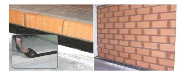
Build the second wall with the same process of the first one and insert the panel in the cavity
