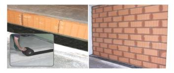
Lay points of a gypsum-based glue on the ground panel or use a low-expansion polyurethane glue
