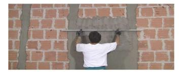
Apply the panel on the wall by forcing with homogeneous pressure
