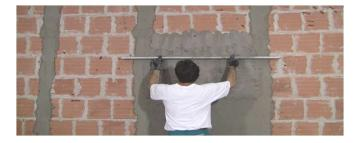
Apply the panel on the wall by forcing with homogeneous pressure
