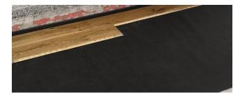
Tape the joints with STIK and glue the flooring on the mat
