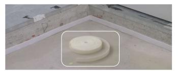
3 Seal the roll jointing borders with Isolgomma Stik tape
