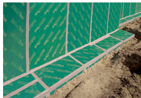
Residential complex foundation, Poland.
