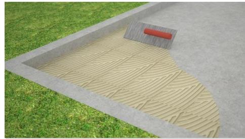
Apply the glue on the concrete surface with a notched trowel of 3 mm
