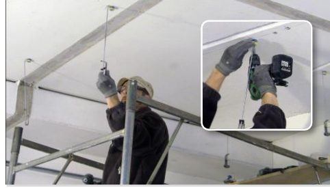
Mark and fix the acoustic hangers
