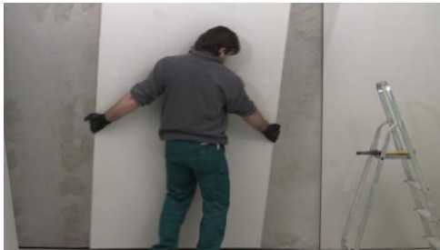
Glue the panel to the wall pressing lightly
