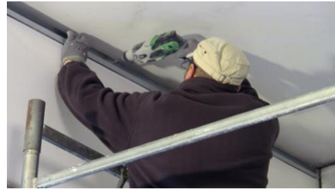
Attach the metal frame along the upper perimeter of the room
