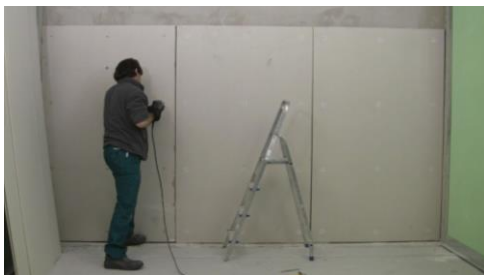
If you do not use the glue, fix the panel with the appropriate plugs
