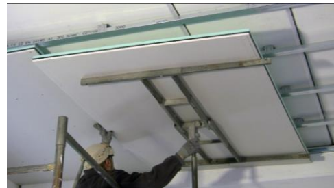
Lean the panel to the metal frame
