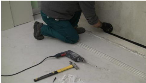
Lay the under wall stripe
