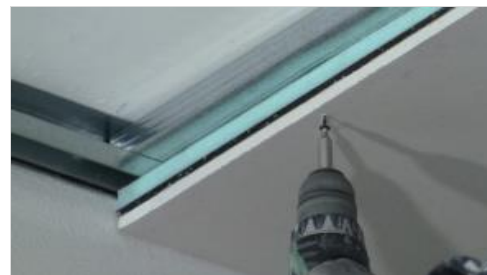
Fix the panel to the metal frame with 55 mm screws every 15 cm
