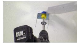
Drill the ceiling e fix the acoustic bracket
