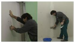
Apply the plastic mesh tape in the gypsum boards jointing lines. Grouting
