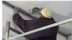
Attach the metal frame along the upper perimeter of the room
