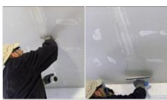
Apply the plastic mesh tape in the gypsum boards jointing lines and grouting
