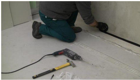
Lay the under wall stripe
