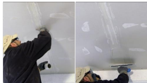
Apply the plastic mesh tape in the gypsum boards jointing lines and grouting
