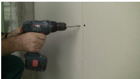
Fix the second gypsum board with the glue and/or appropriate screws
