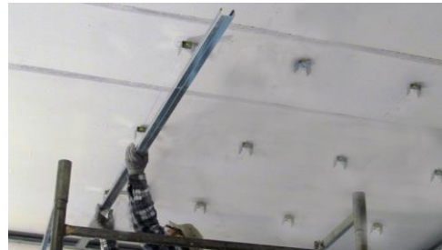
Fix the metal stud to the acoustic bracket
