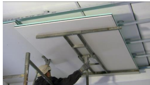
Lean the panel to the metal frame
