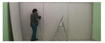
Apply the plastic mesh tape in the gypsum boards jointing lines. Grouting
