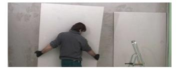
Fix the second gypsum board with the glue and/or appropriate screws
